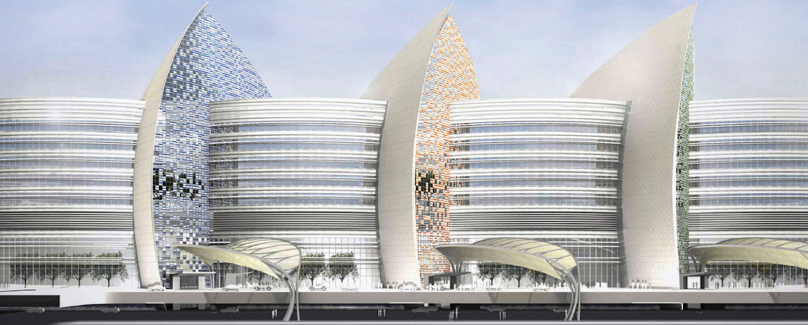
Sidra Hospital Doha, Qatar M&E Consultant KEO International
