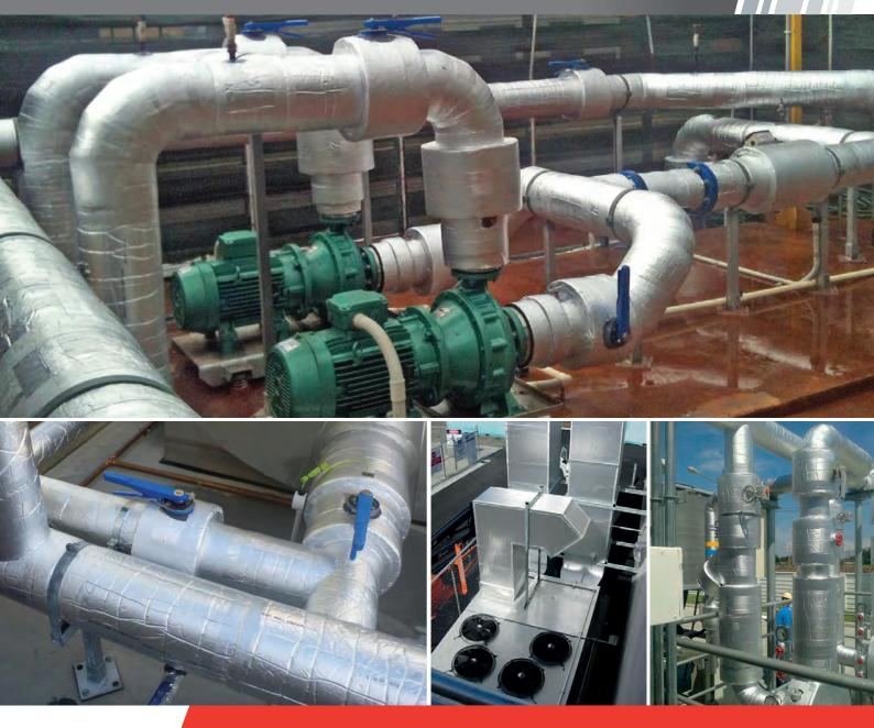
Closed cell, physically crosslinked polyolefin foam insulation with ultra tough foil facing to prevent mechanical damage in high risk areas.
